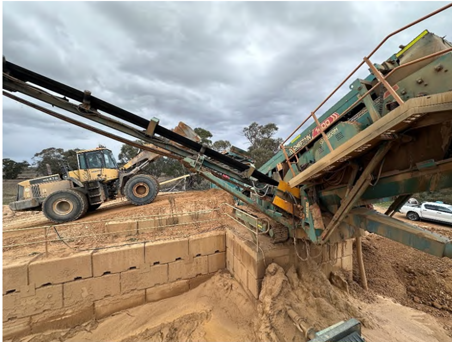
Figure 17: Wet Screen plant on Site
